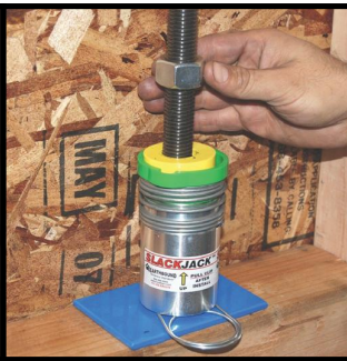
Place colour coded washer and spin nut down hand tight.
