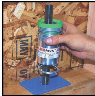
Slide Slackjack® on top of colour bearing plate.
